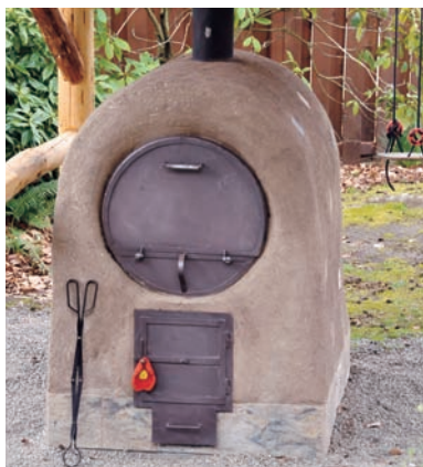
A Barrel Oven made with red brick and finished with an earthen plaster. (Photo, June Bonnheim)
