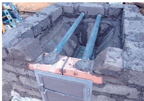
8. Bricks, Firebox, Lintels
