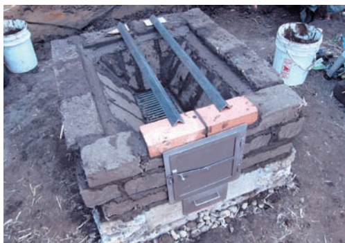
7. Bricks, Firebox, Lintels
