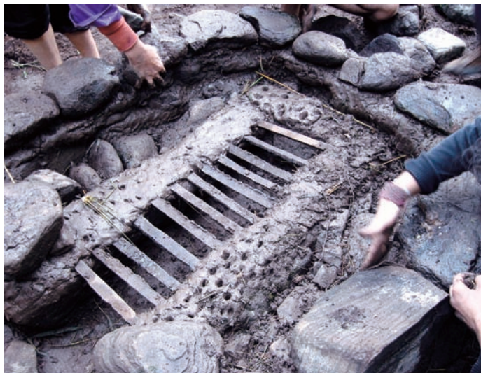
Though you can use recycled pieces of metal and embed them in cob, we have found that this is not so durable over time.
