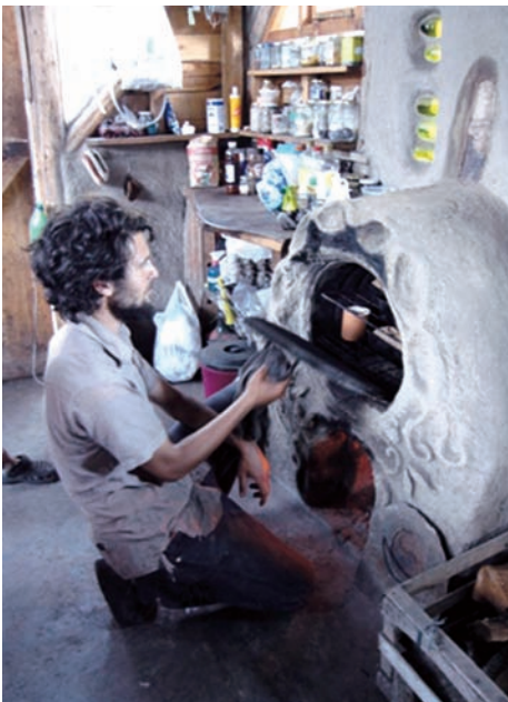
The face of a Barrel Oven can be built inside a building while the bulk of its body and the chimney remain outside.
