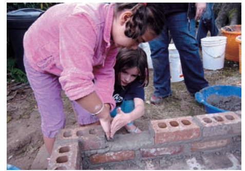
Common red brick are great to build with and easy to find, often for free. Mortar made from clay and sand is enjoyable to apply by hand.
