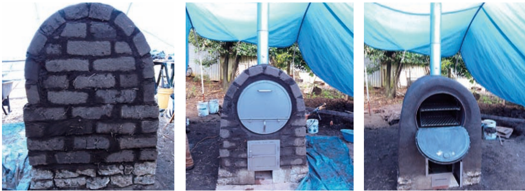
15. Shaping and Rough Plaster
