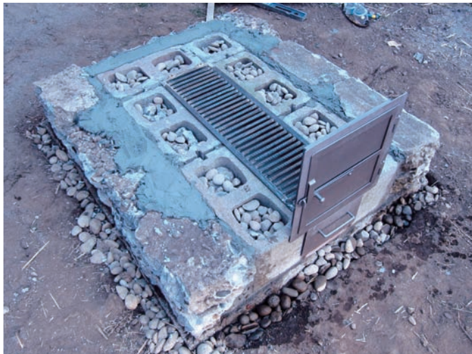
The grate sits upon the ash space you have created. Here you can see a durable grate and firebox door made by Firespeaking.
